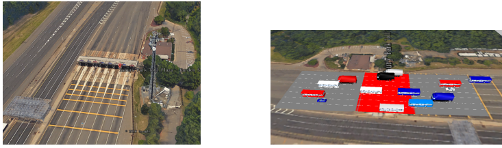
Figure 12: Asbury Toll Plaza
